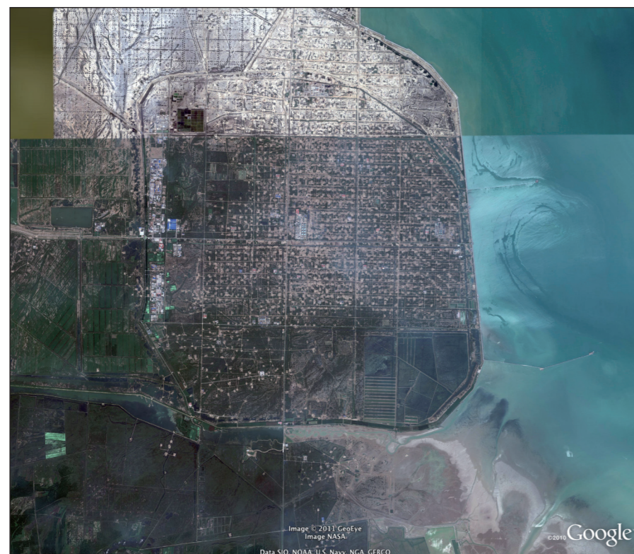
Figure 1: GEO-EYE satellite image of the Yellow River (Huanghe) delta. Each year 33.6 Mt of crude oil are extracted from the delta. The Gudong Seawall, built 1985-1988 to protect the oil fields from inundation, is 10 m thick at its top and 38 m at its bottom. The oil rigs are laid out on a grid pattern. The field is presently below sea level by 1 to 2 m, protected from the sea by the Seawall. Image from Google Earth Pro; pixel resolution is ~1 m.
